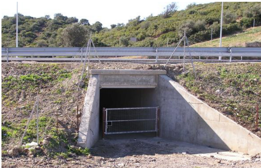
Figure 5.15. Unforeseen human uses must be identified and corrected during maintenance. In this case, a farmer installed a gate to prevent his sheep from using a wildlife underpass. Photo: Luis Ramajo / Junta de Andalucía.
