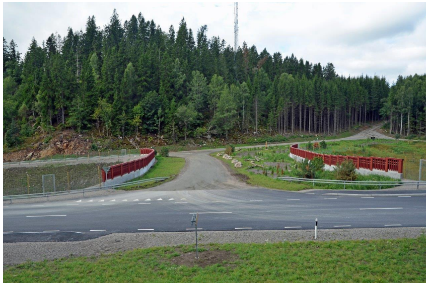
Figure 5.16. Multi-use overpasses require the maintenance of screens, fences, vegetation and refuges, but also other factors related to traffic and human uses. Photo: Mats Lindqvist.
