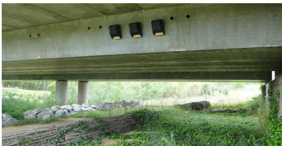
Figure 5.14. Woodpiles, dry stone walls and bat refuges installed under a viaduct. All of them require adapted maintenance tasks to ensure their long-term conservation. Photo: Minuartia.
