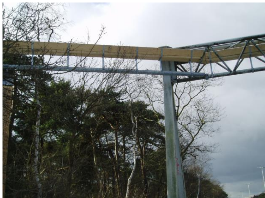
Figure 5.17. Canopy bridges require the maintenance of wooden structures that provide passages for arboreal mammals. Photo: Hans Bekker.
