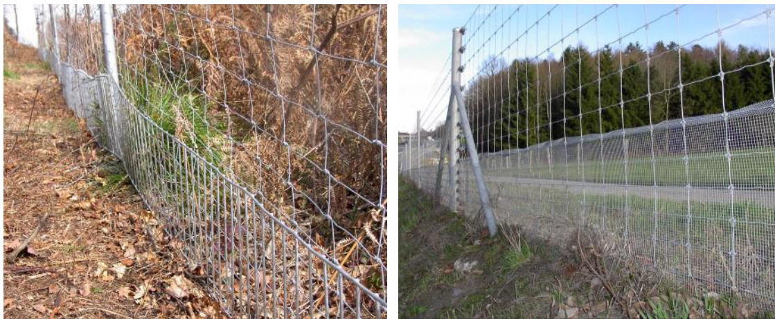
Figure 5.10. Wire mesh fences could be reinforced to stop specific target species from entering. On the left is specific reinforcement that is resistant to wild boar; on the right, reinforcement for small fauna. Photos: Carme Rosell.
