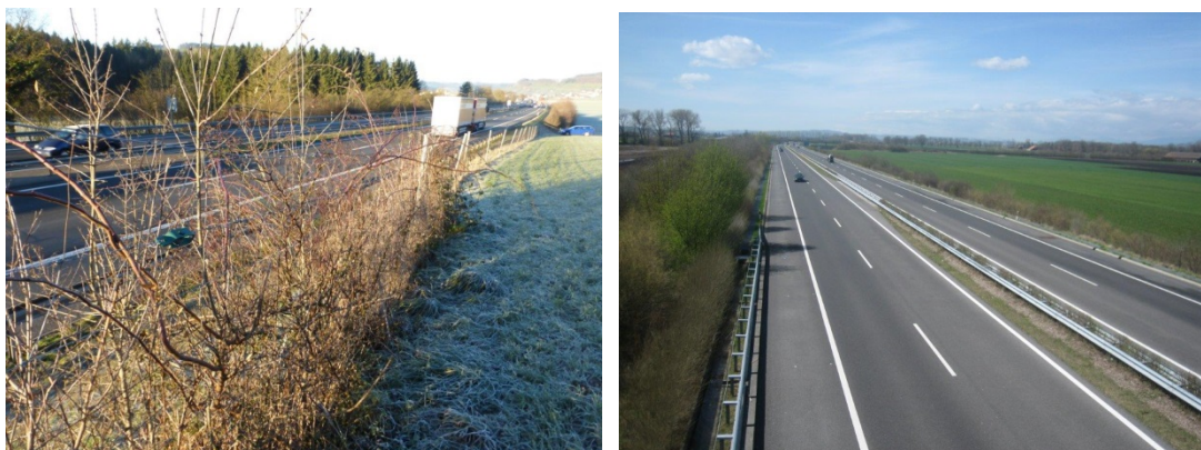
Figure 5.6. In open landscapes such as meadows and cropland the outer hedge may reinforce the function of the fence, making it more difficult for deer to jump or boar to breach it (at left). It can also create a corridor along the road guiding the animals towards wildlife crossings and reducing dispersal of pollutants or other disturbance. Photo: Marguerite Trocmé.
