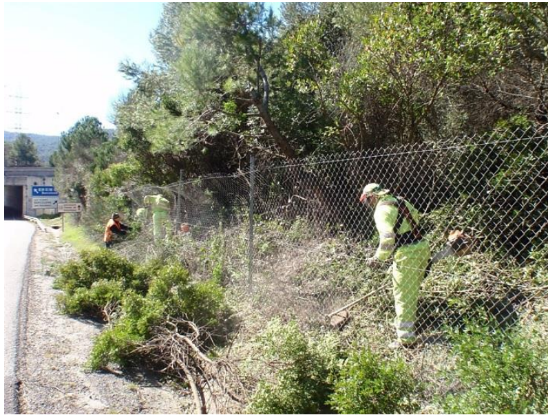
Figure 5.5. Mowing and pruning of a corridor along the fence in sections crossing dense forests or bushes will reduce damage to mesh and facilitate fence maintenance tasks. Photo: Tunels de Barcelona-Cadí.
