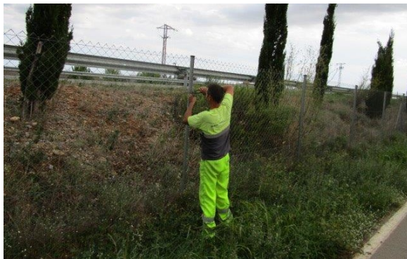
Figure 5.4. Anchoring the mesh to the poles and repairing mesh damaged by wildlife are important to reduce the risks of wildlife-animal collisions. Photo: Department of Territory and Sustainability, Catalan Government.
