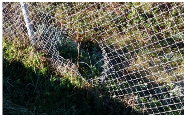
Figure 5.4. Anchoring the mesh to the poles and repairing mesh damaged by wildlife are important to reduce the risks of wildlife-animal collisions. Photo: Department of Territory and Sustainability, Catalan Government.
