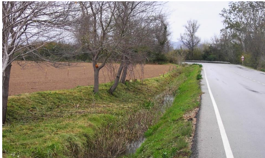
Figure 5.26. Road verge management may be adapted to several functions. In this case, an area has been cleared of shrubs to reduce the risk of wild boar-vehicle collisions. Photo: Carme Rosell.
