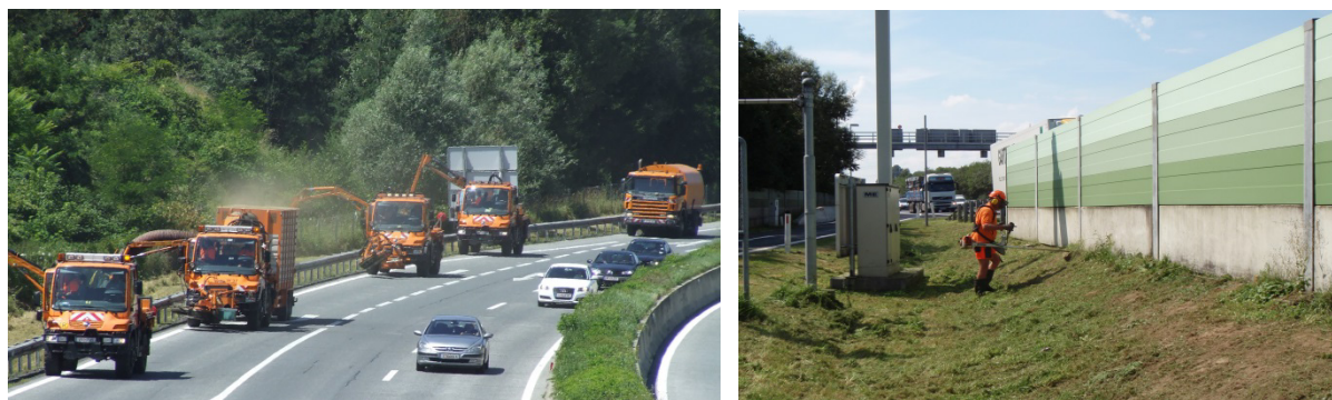
Figure 5.23. On the left: trucks equipped with different tools working at the same time to cut strips of vegetation at different heights and to remove mowing debris. On the right: in sensitive places, manual mowing could be done. Photo: ASFINAG.
