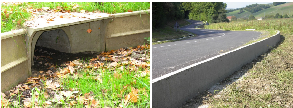
Figure 5.8. Amphibian guiding fences could be made from concrete, metal or polymeric materials and maintenance should be adapted appropriately. A corridor along the fence must be kept free from obstacles. Photo: Miklos Puky (left); Carme Rosell (right).
