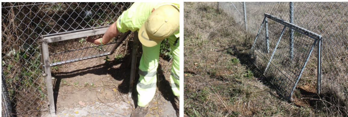
Figure 5.7. Escape gates require high maintenance and frequent inspection to guarantee proper functionality and ensure that they do not remain open as wildlife could use them to enter the fenced area. Photo: Tunnels of Barcelona-Cad ; Joana Colomer (right).
