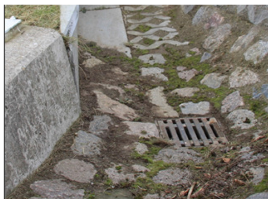
Figure 5.9. Inspections should detect ecological traps such as gullies beside fences for small fauna. Proper solutions must be provided to prevent the accidental fall of animals. Photo: Heinrich Reck.
