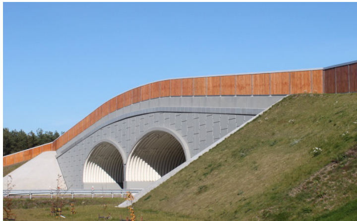
Figure 5.3. Screen maintenance must guarantee perfect continuity with fences and other road elements. Photo: Carme Rosell
