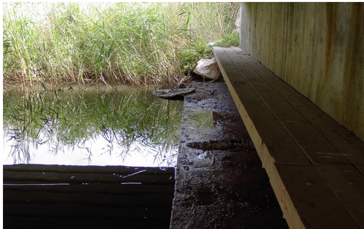
Figure 5.28. Modified culverts require proper inspections and removal of any obstacle (branches, rocks, debris, etc.) that hinder the movements of fauna. Dry ledges could be located on culverts during road operation to improve their function as wildlife crossings. Photo: Minuartia.
