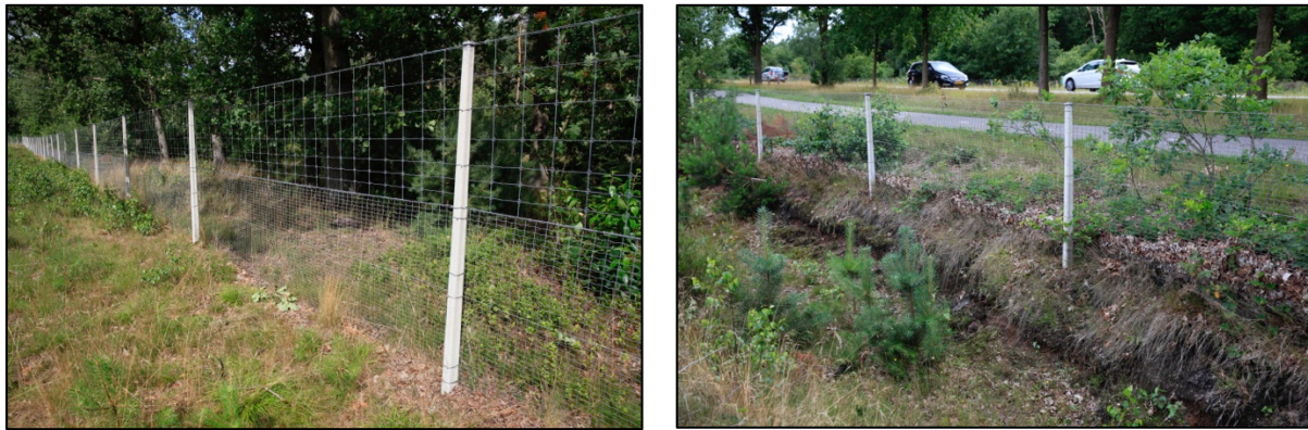
Figure 3.3 Wildlife exclusion barriers along highway N227: two-metre high wildlife fences without a ditch (left) and one-metre high wildlife fences in combination with a one-metre deep ditch with a steep edge on the side of the road (right).
